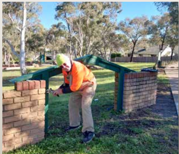
The new sign being installed by Kim. The six missing half bricks will also be attended to with the assistance of another member Ken McLean.
