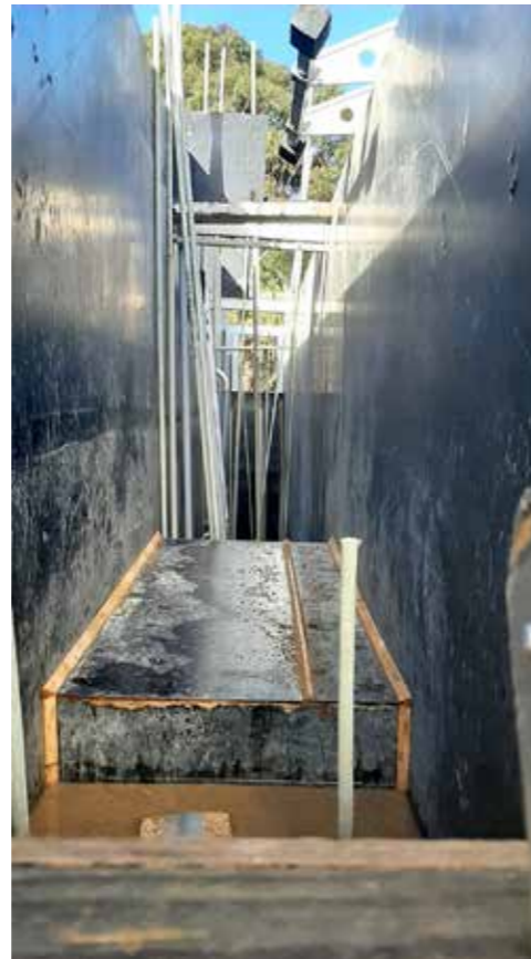
↑ Inside the formwork: not for the faint hearted or claustrophobic.
