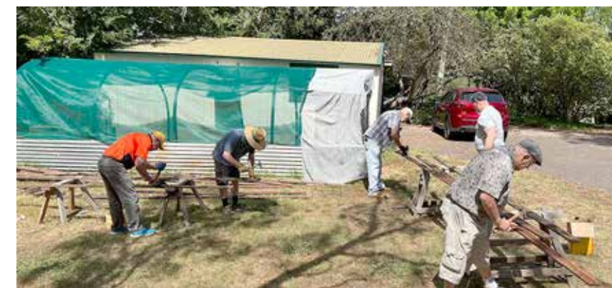
De-nailing the decking boards for the deck.
