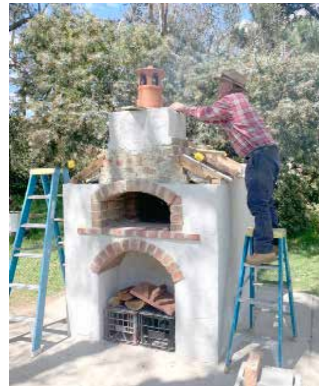
Dennis doing a test fit of the chimney top.
