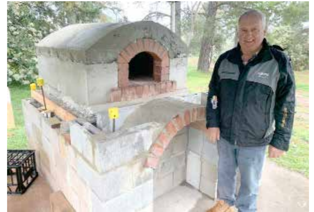
Dennis next to the internal brick/concrete skin of the oven, prior to more insulation and the outer skin being added.
