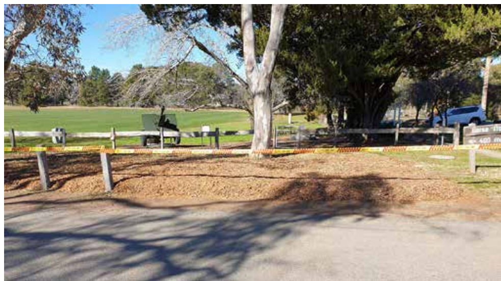
Mulch laid in preparation for bollards to be replaced.
