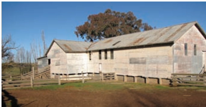
The old Gold Creek shearing shed
