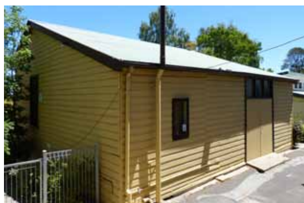
7.21 (5) South/East elevation (dated 2014)
