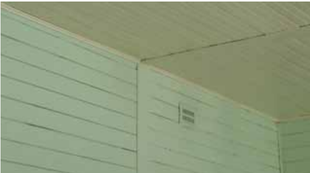
7.22 (9) Original weatherboard lining
