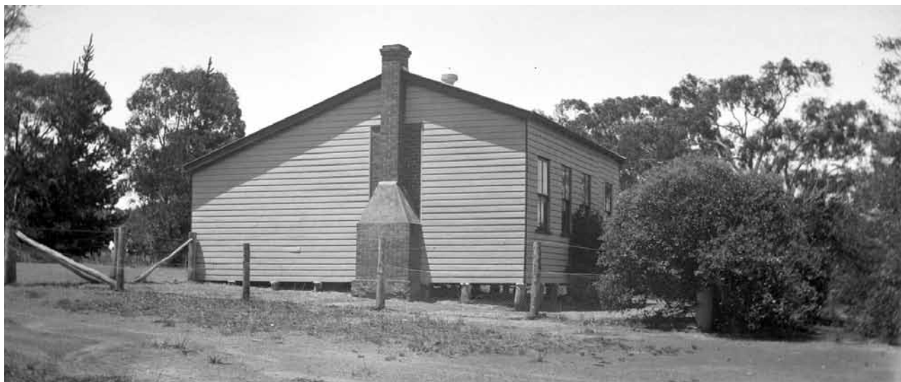
6.5 (2) The extended building with enclosed playground
