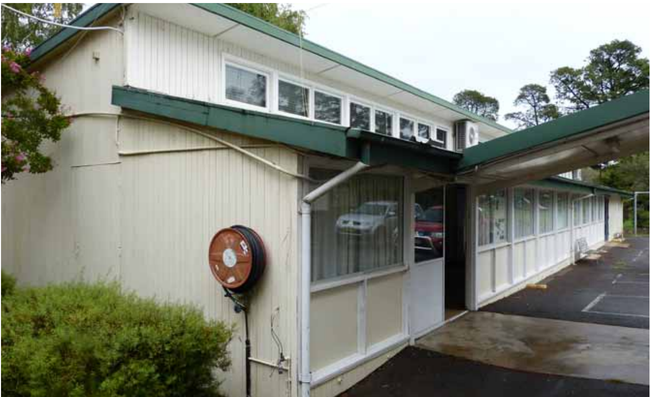
11.0 (1) The building erected in 1960 and extended in 1967 (photo 2014)
